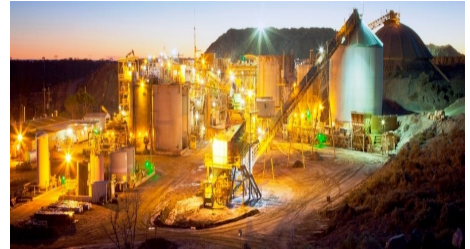
1.2 million tpa CIL Plant
