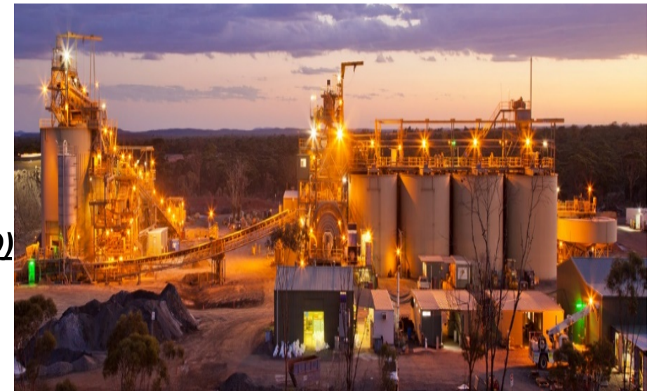
1.3 million tpa CIL Plant 12
