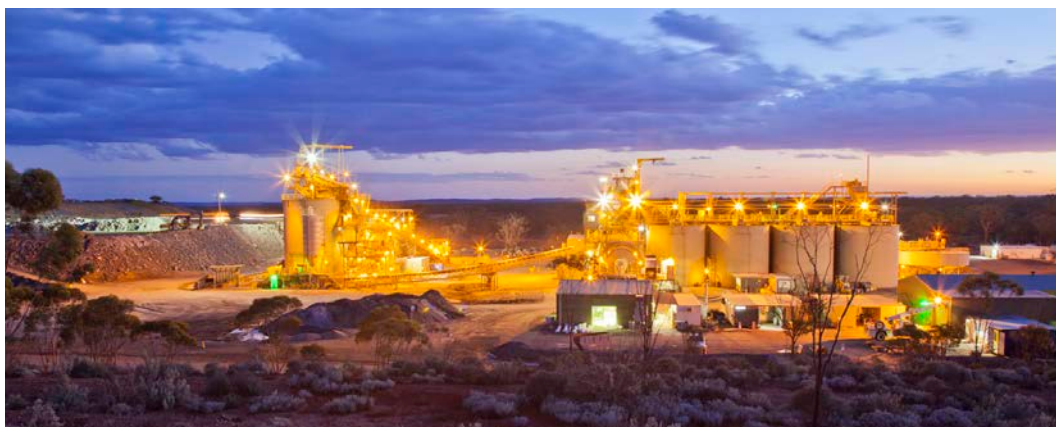
HGO Processing Facility
