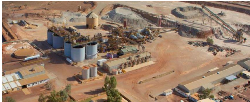
Bluebird CIP Plant – 1.8mtpa
