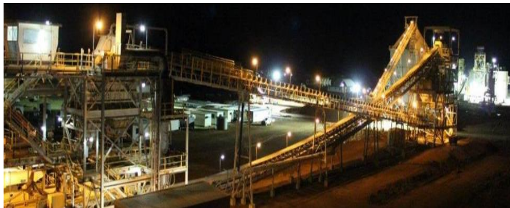
Tuckabianna CIP Plant – 1.8mtpa
