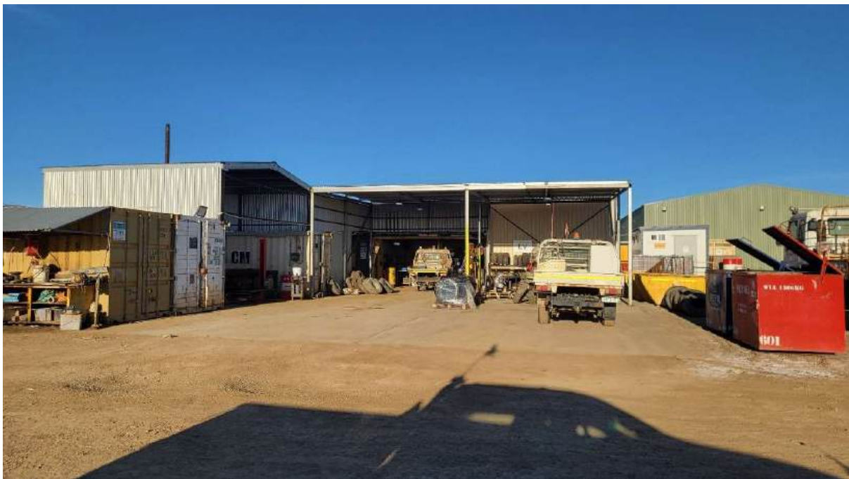
Figure 18-3 Big Bell light vehicle workshops - Source: Westgold.
