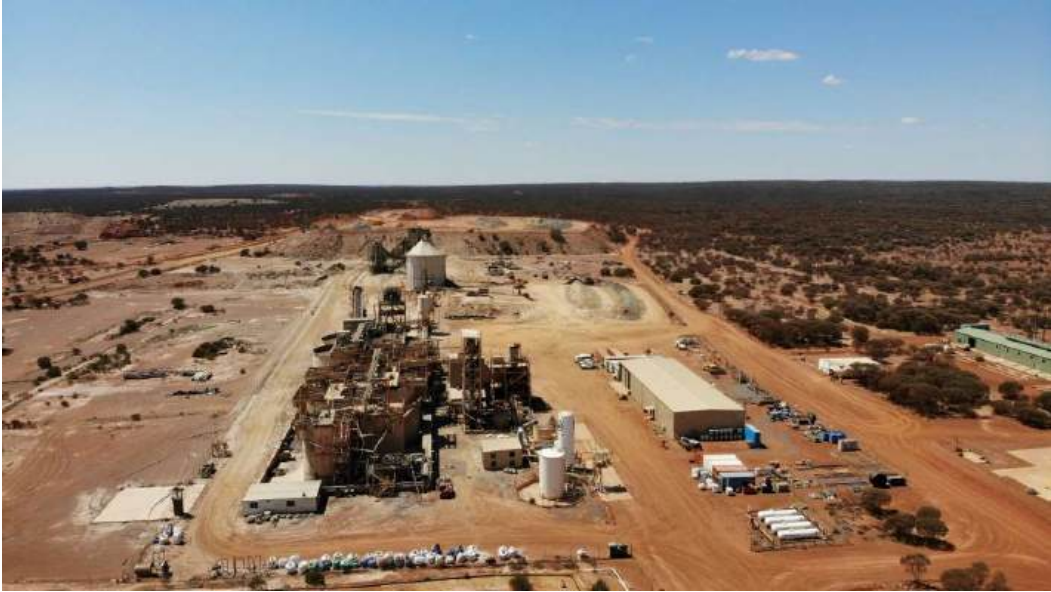
Figure 18-4 Tuckabianna mill and workshops - Source: Westgold.
