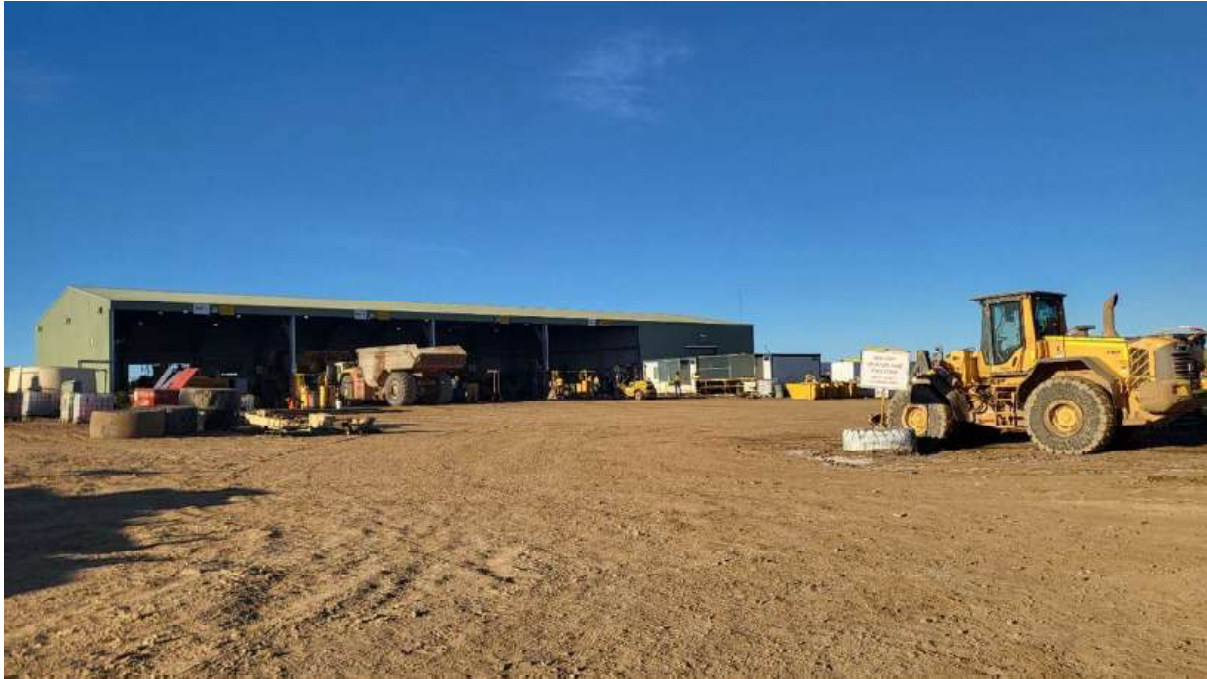
Figure 18-2 Big Bell heavy vehicle workshops - Source: Westgold.
