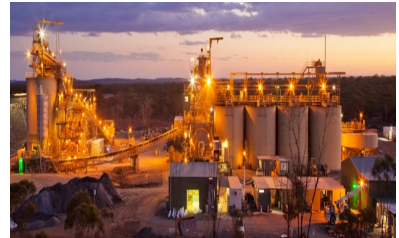
1.3 million tpa CIL Plant
