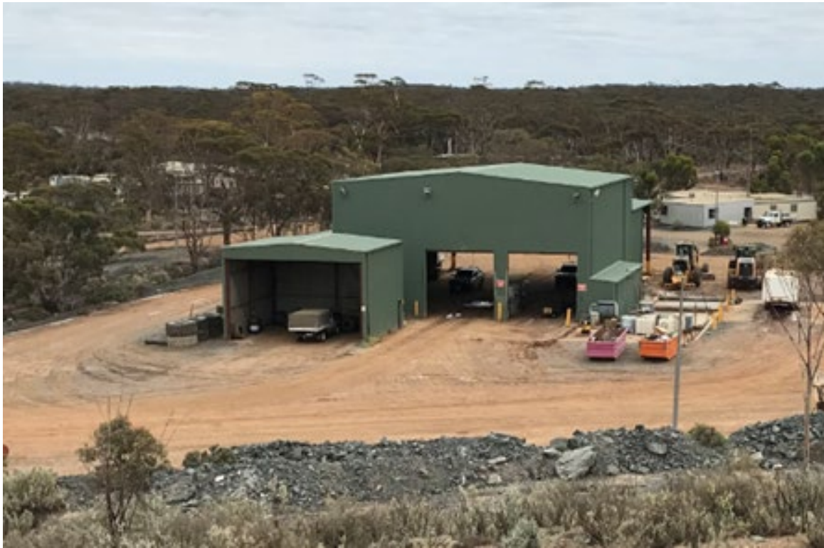
Figure 18-4 HGO underground workshop – Source : Westgold.
