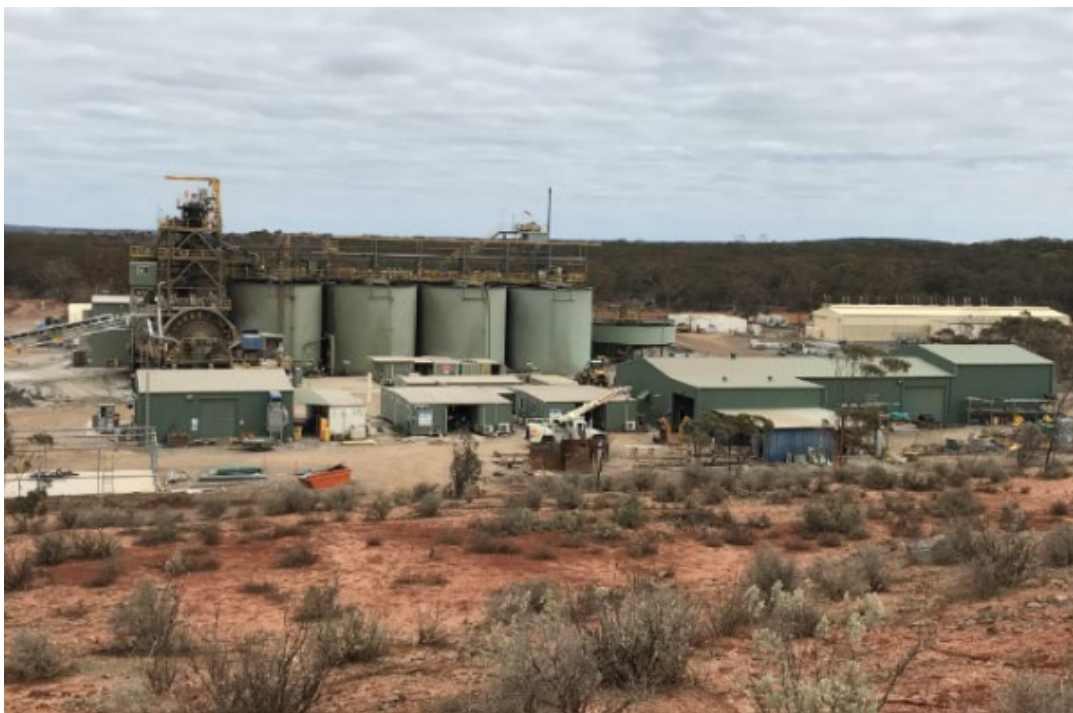
Figure 18-6 Higginsville processing plant and workshop/store – Source : Westgold.
