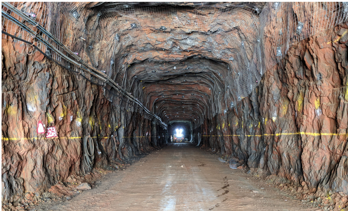
Looking down the rehabilitated Big Bell decline.
