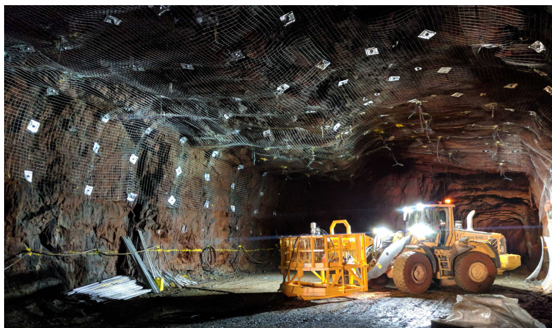
Rehabilitation of the truck passing bay in the Big Bell decline.
