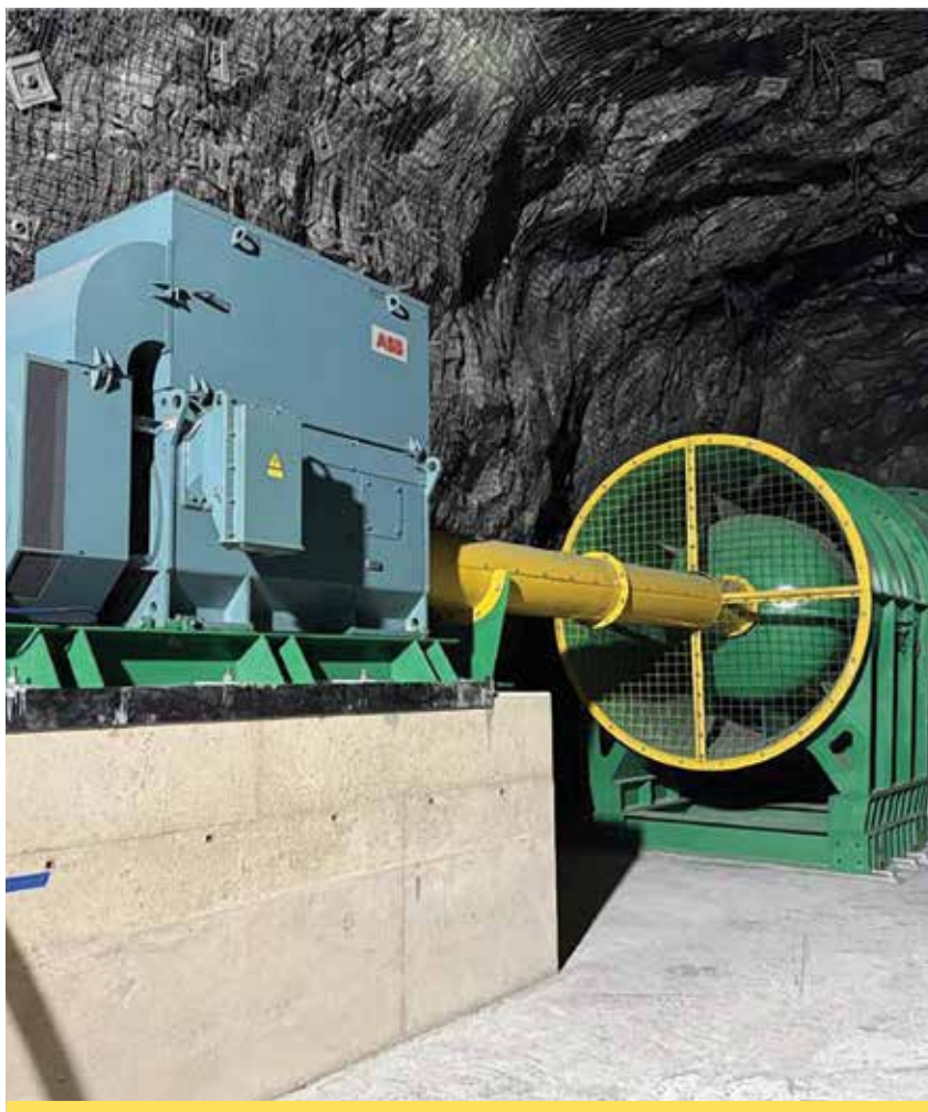
Beta Hunt Infrastructure Upgrade
