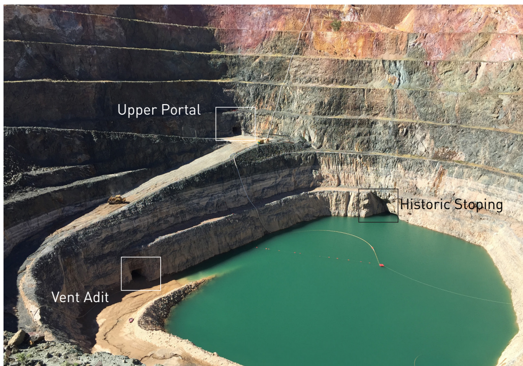
Starlight Pit - Exposed Portals and Stope Void
