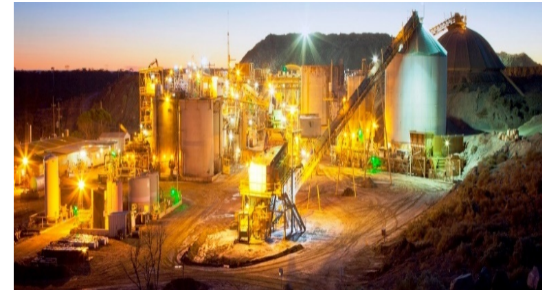
1.2 million tpa CIL Plant
