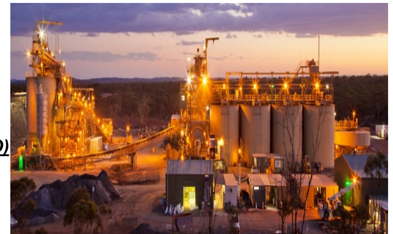
1.3 million tpa CIL Plant
