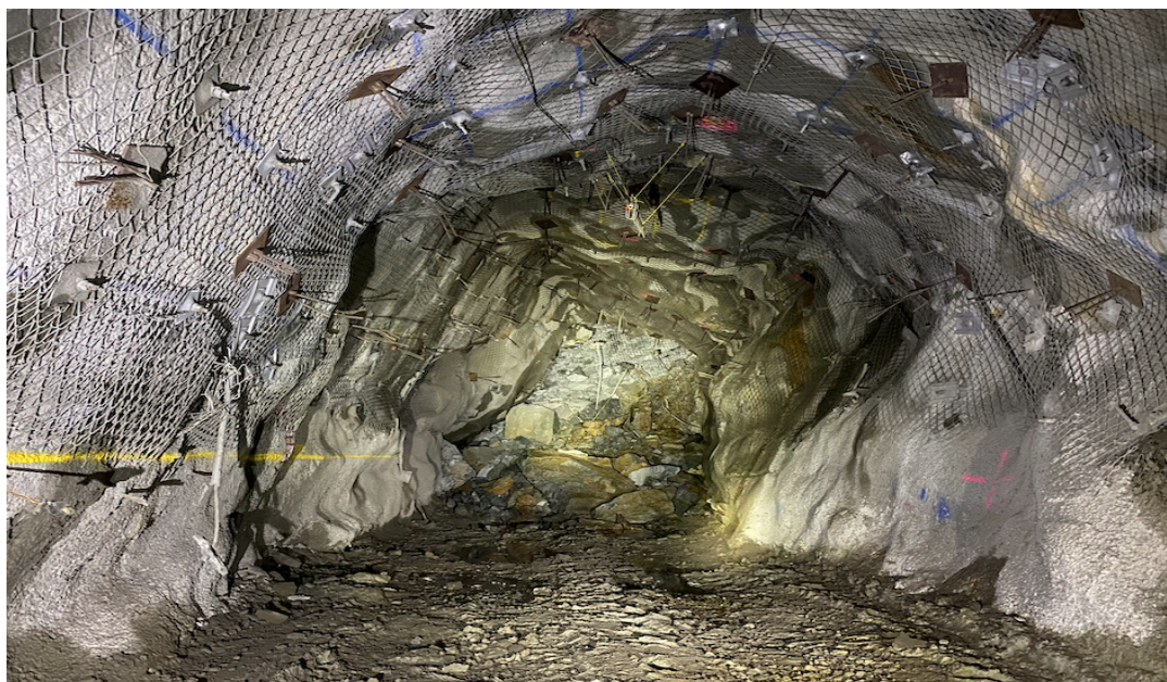
Figure 6: Image showing 560 Ore Drive and drawpoint after mass blast.
