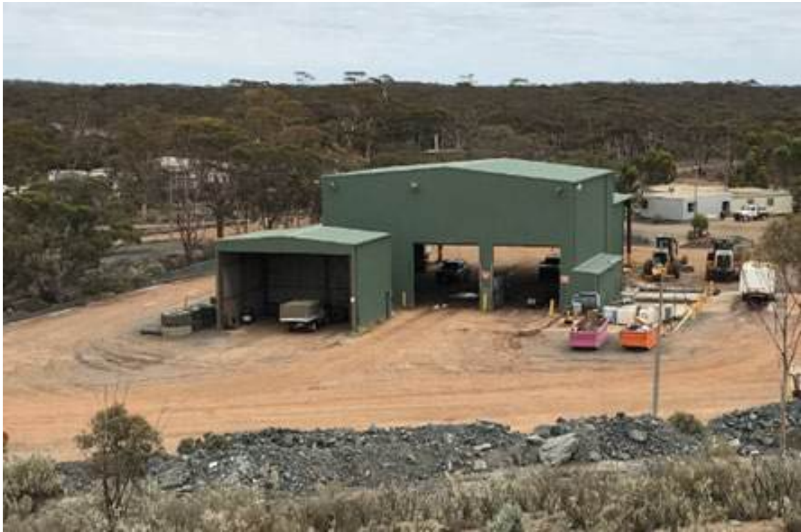
Figure 18-4 HGO underground workshop – Source : Westgold.
