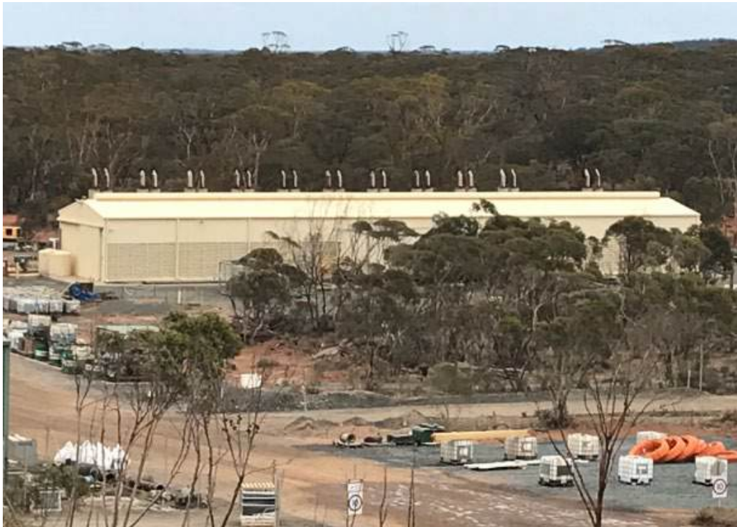
Figure 18-3 HGO powerhouse – Source : Westgold.
