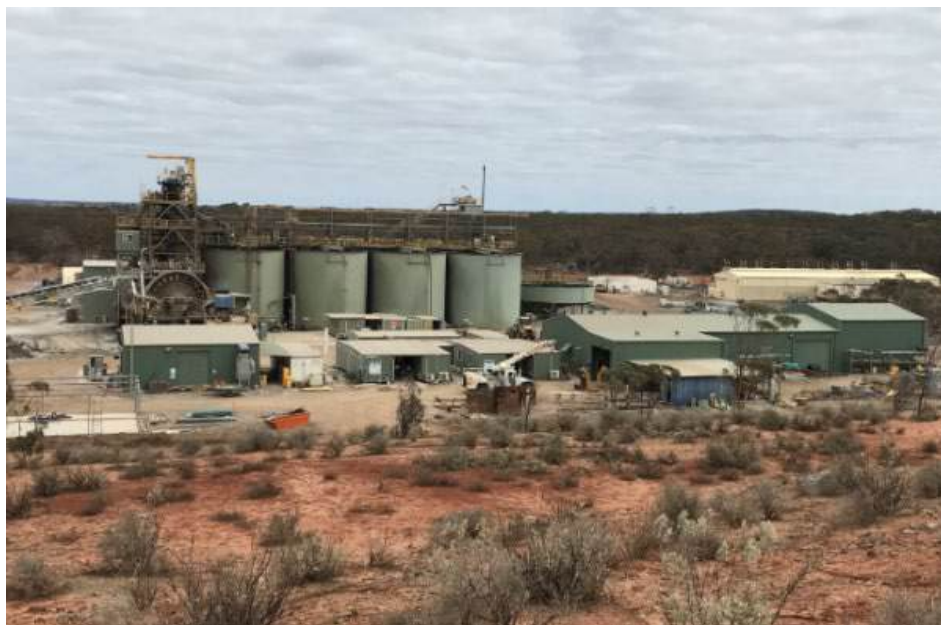
Figure 18-6 Higginsville processing plant and workshop/store – Source : Westgold.
