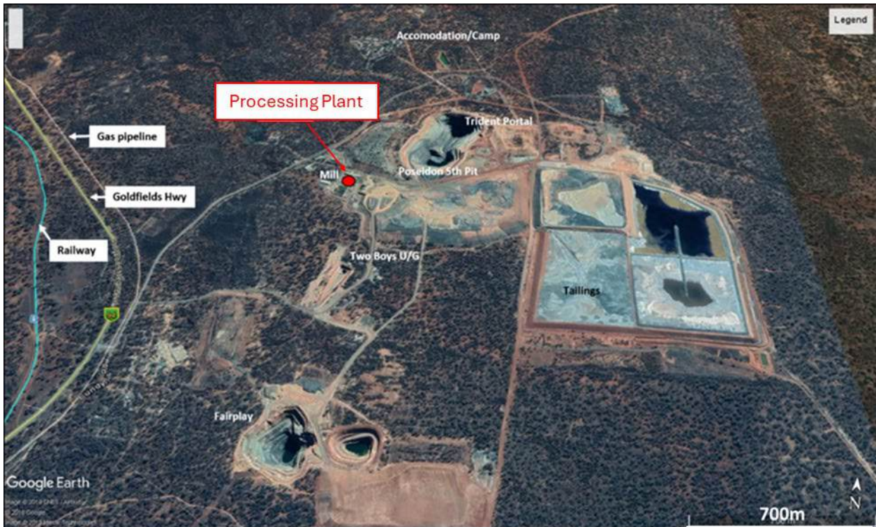
Figure 5-2: Higginsville processing plant – oblique aerial view. Shows the access to the Higginsville processing plant and offices via a constructed all-weather access road (0.8 km) from the Goldfields Highway – Source : Westgold.
