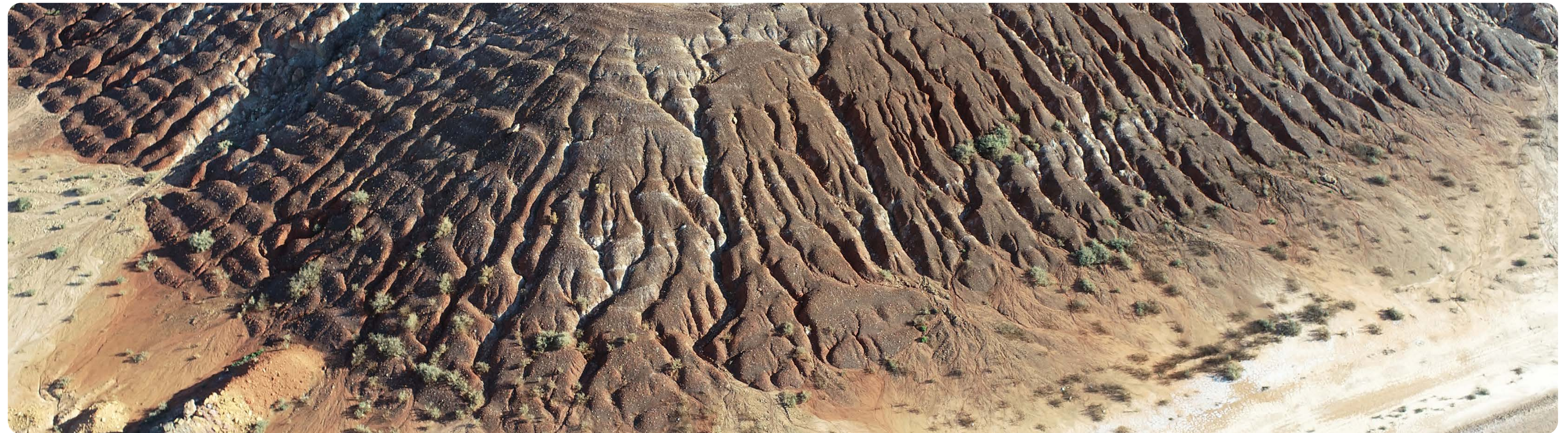
Erosion on the Black Swan South WRD (constructed 1999-2006)
