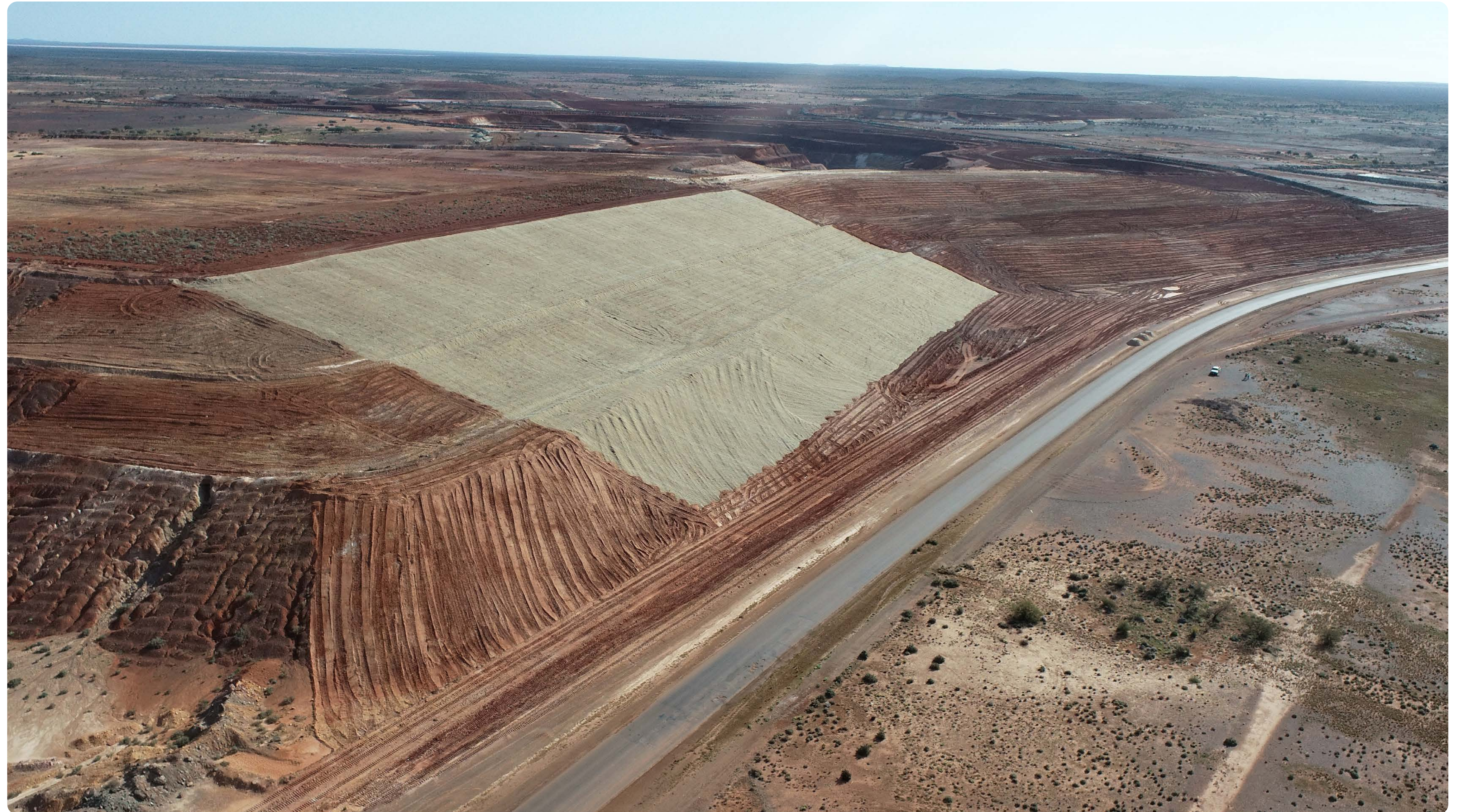
Installation of Jute Matting on Black Swan South WRD
