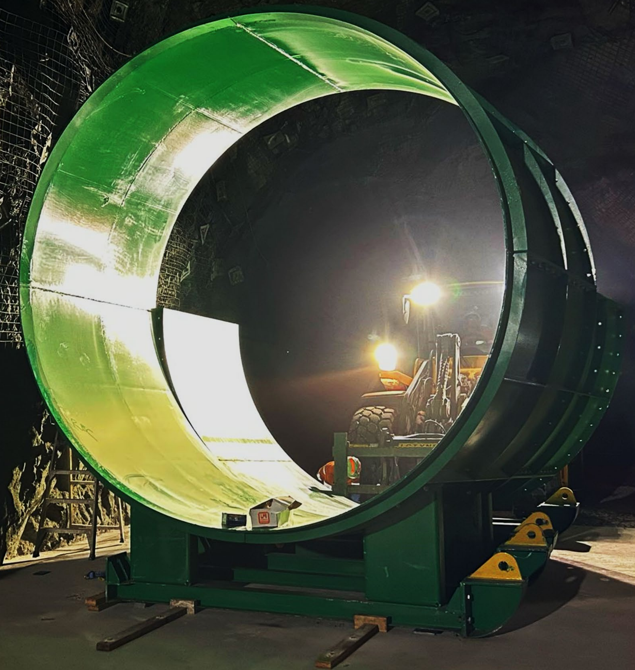
Installation of primary fan upgrade in early April 2025
