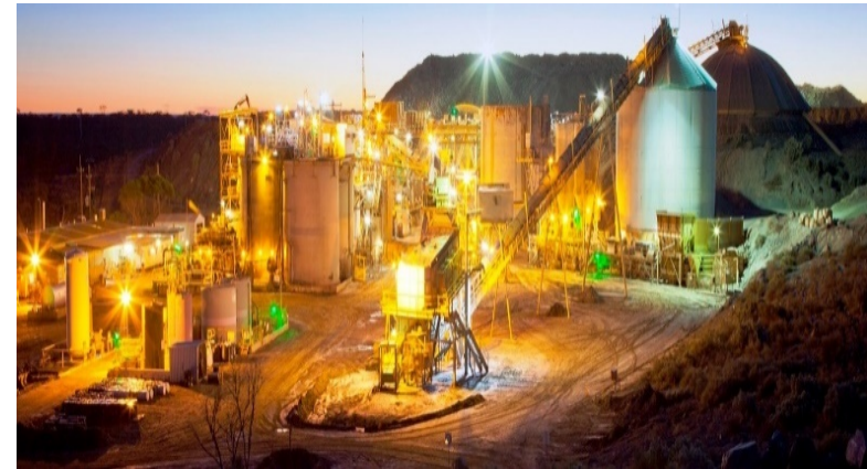
Jubilee Plant - 1.2 million tpa CIL
