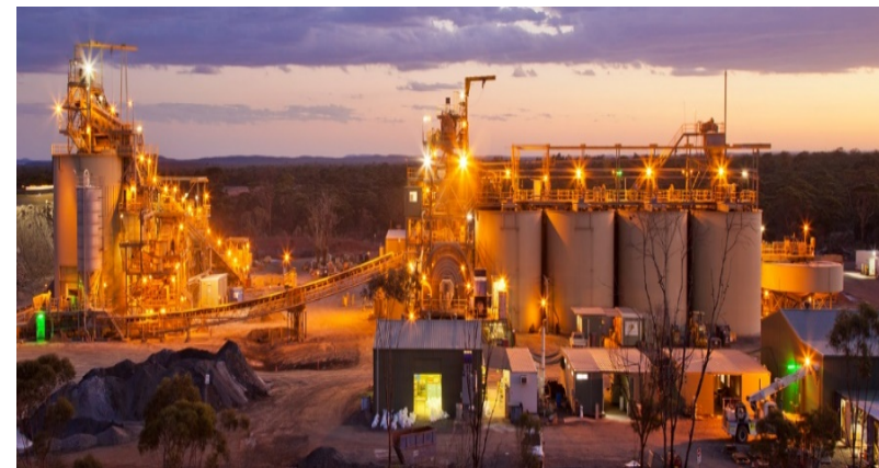
Higginsville Plant - 1.3 million tpa CIL
