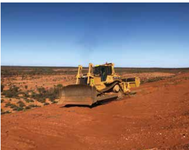
Progressive rehabilitation ripping and seeding waste rock dump
