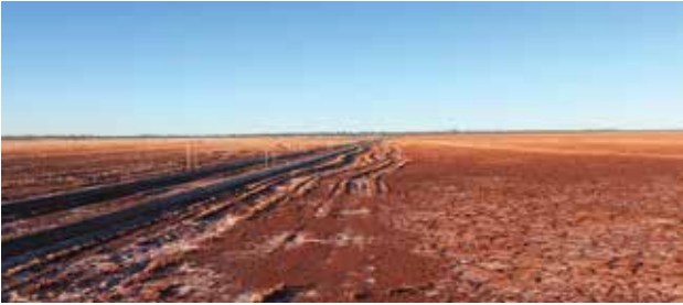
Dewatering to Lake Austin
