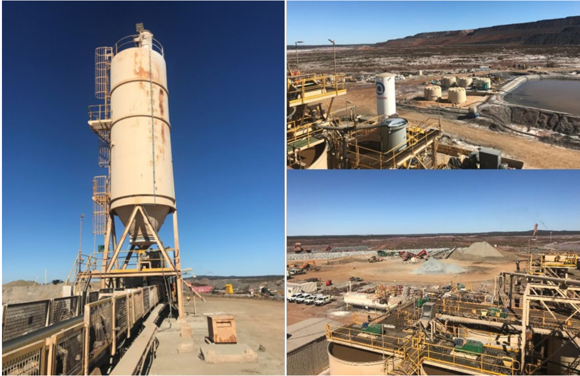
Figure 6-4 Lakewood processing plant (2022) – Source : Westgold.
