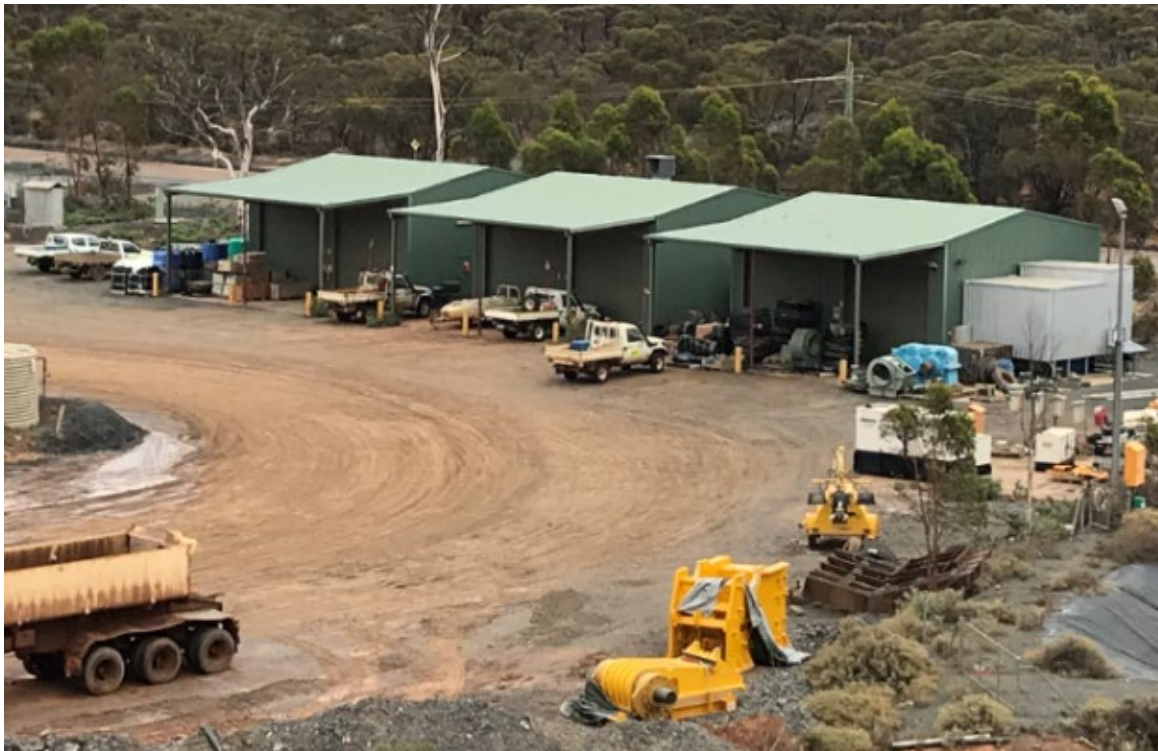
Figure 18-5 HGO light vehicle workshops – Source : Westgold.
