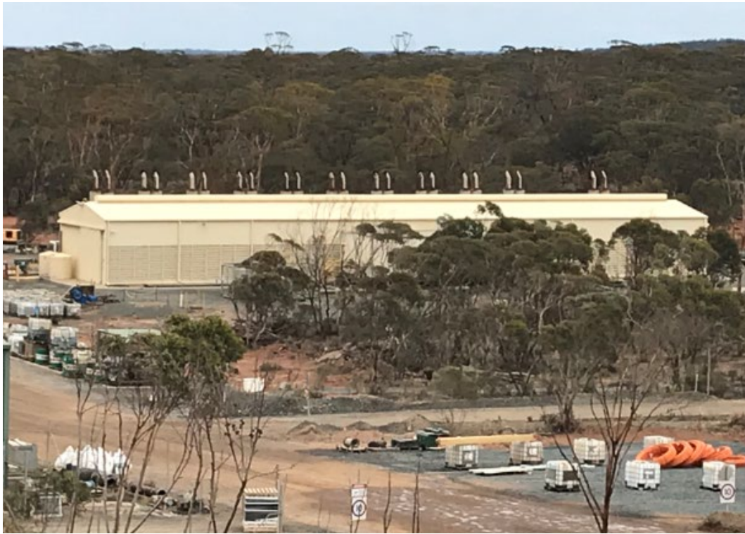
Figure 18-3 HGO powerhouse – Source : Westgold.
