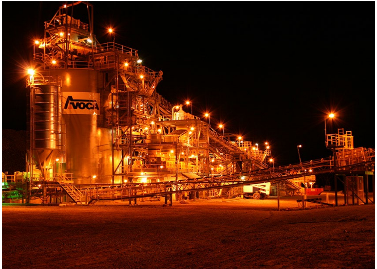
Figure 6-3 Higginsville processing plant (2008) – Source : Westgold.
