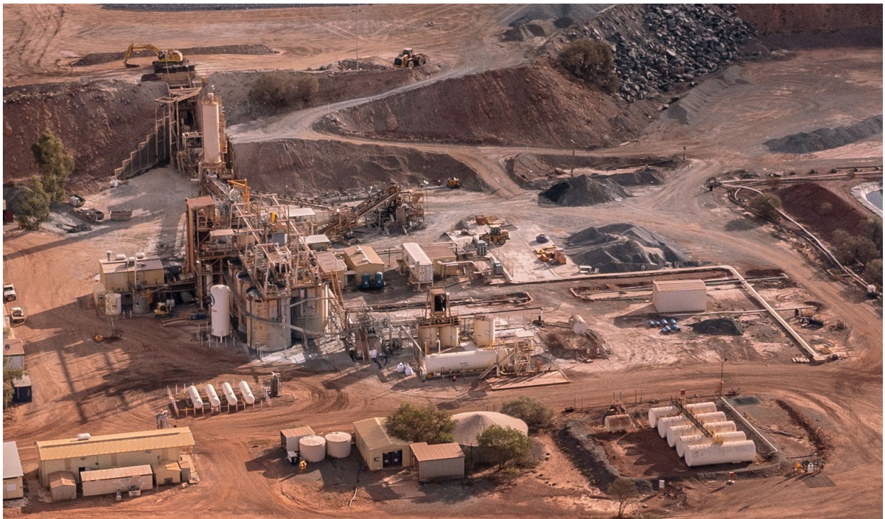
Figure 2 – Fortnum Processing Plant
