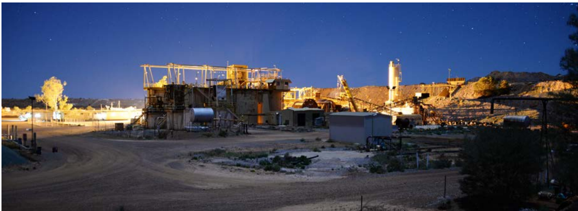
FGP Processing Facility
