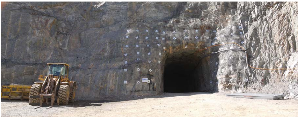
Starlight Underground Mine Portal
