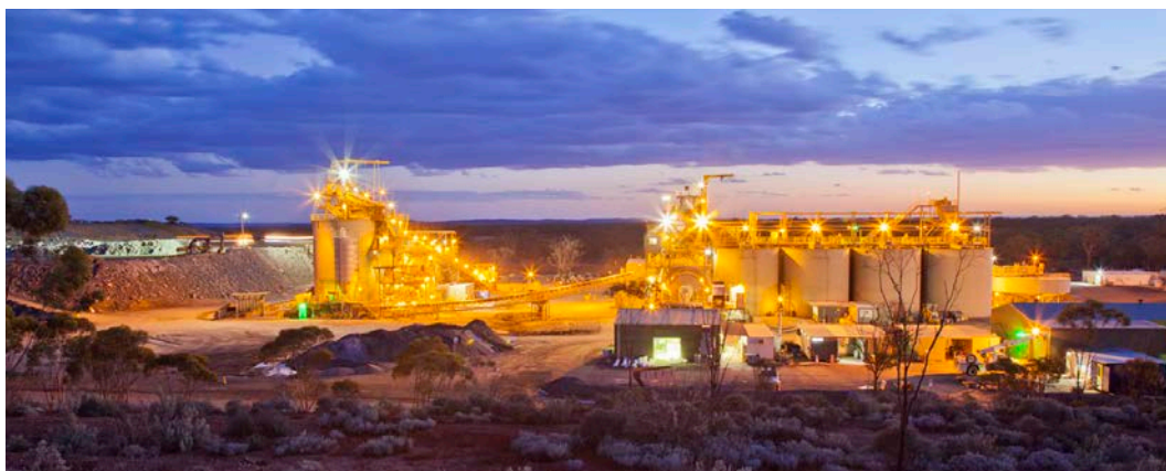
HGO Processing Facility
